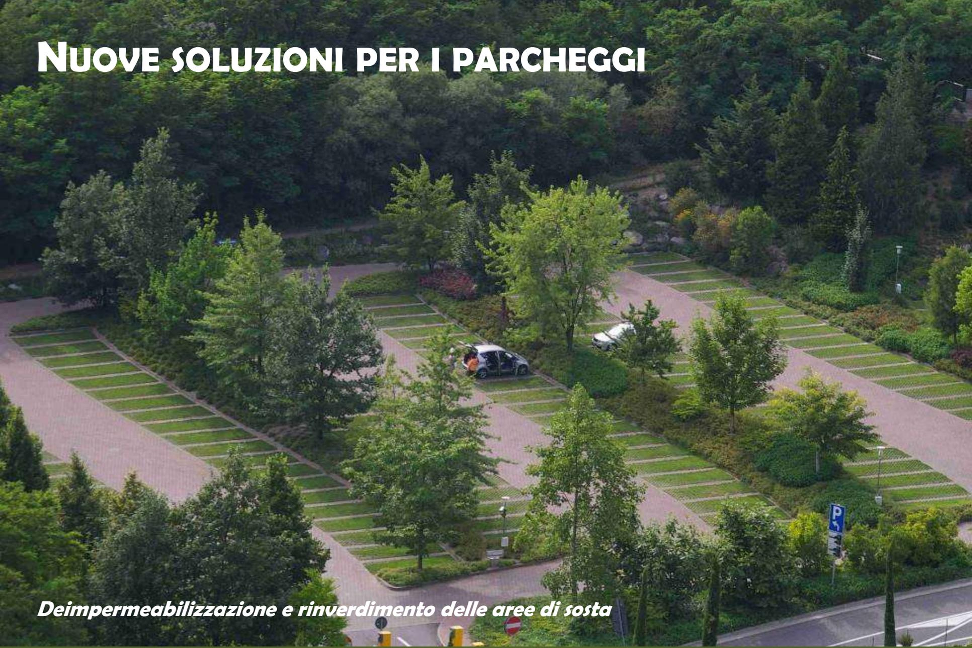
An aerial photograph of a parking lot designed with permeable paving and integrated greenery. The parking spaces are separated by light-colored, textured paving stones, and the areas between them are filled with green grass. The lot is surrounded by numerous trees and shrubs, creating a lush, natural environment. A few cars are parked in the lot, and a blue parking sign is visible in the lower right corner. The background shows a dense forest on a hillside.
